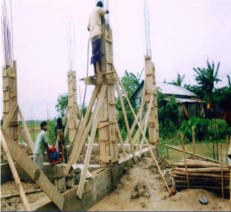
Construction of Columns
