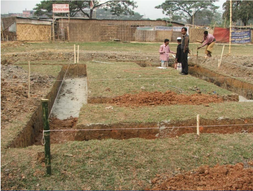
Giving layout Trench cutting
