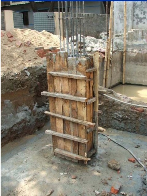
Column casting up to grade beam
