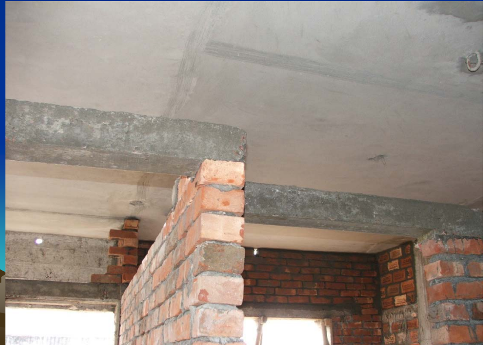
Construction of Lintels
